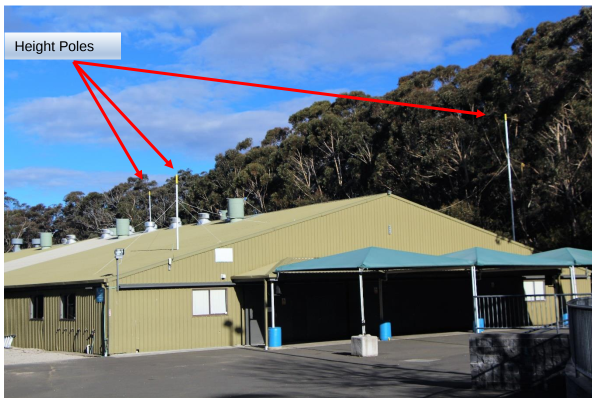
Figure 6 View of auditorium with height poles
