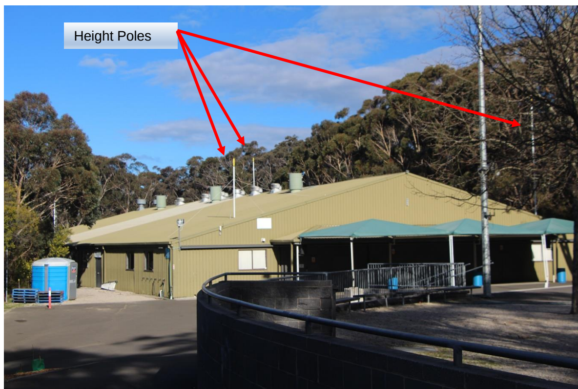
Figure 5 View of auditorium with height poles
